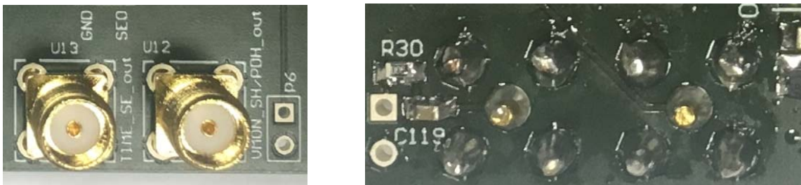
Figure 9: (left) TIME_SE_out and VMON_SH/PDH_out outputs; (right) location of the C119 capacitor for the Accoupling of shaper/PDH signal.
